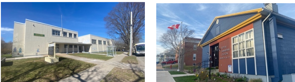
Figure 10. Halifax Inglis Street Junior High School and Lunenburg Royal Canadian Legion Building (Photos by Durgun Şahin, 2022)
