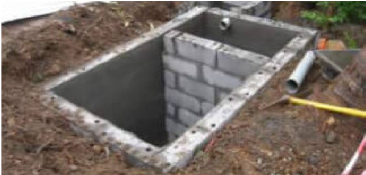
Figure 2: A conventional septic system in rural areas
