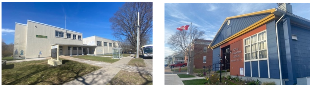
Figure 10. Halifax Inglis Street Junior High School and Lunenburg Royal Canadian Legion Building (Photos by Durgun Şahin, 2022)
