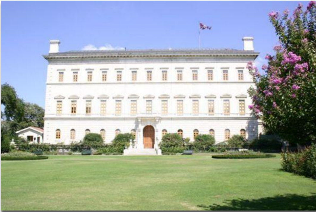
Figure 1. British Embassy in Istanbul (Arup Archive)
