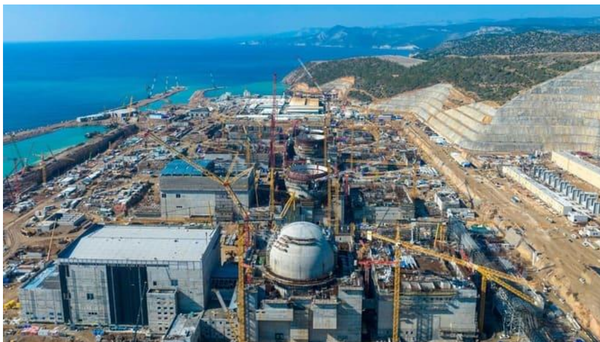
Figure 1. An image of the Akkuyu Nuclear Power Plant construction
