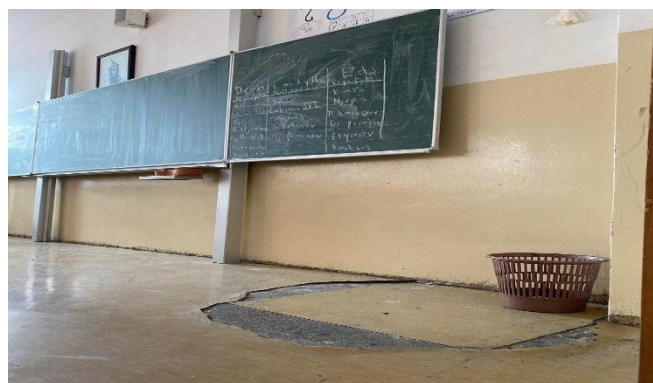
Figure 5. Damaged floor
