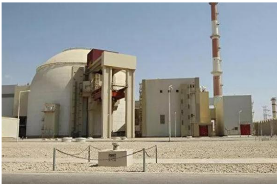
Figure 4. Hydrogeological monitoring well at the Bushehr-1 NPP site
